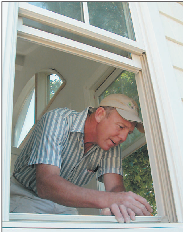
Scott Cronshaw of Cronshaw Carpentry marks the cuts for a piece of window casing to be used in the remodel of a house in Oxford.
